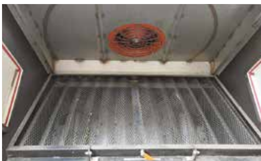
Inside the Minor 25 hopper
