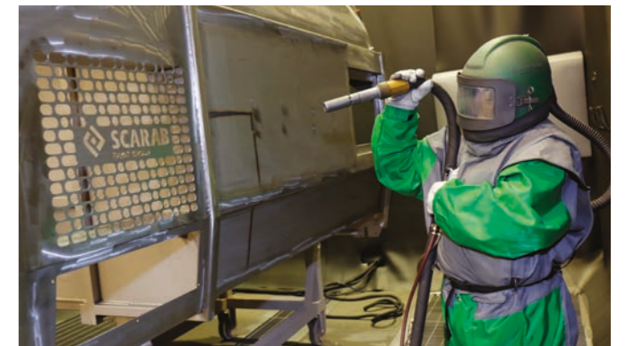
Shot blasting the stainless steel hopper
