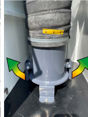
Open sprung clips to release from blanking plate
